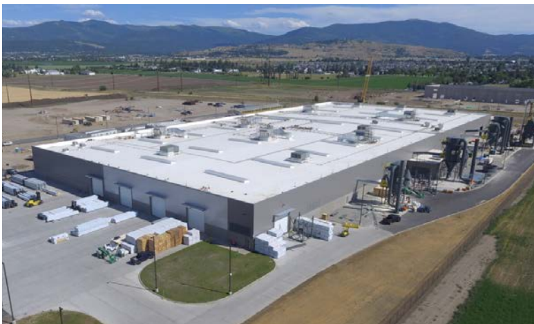
Spokane Valley Mass Timber Factory Tour
